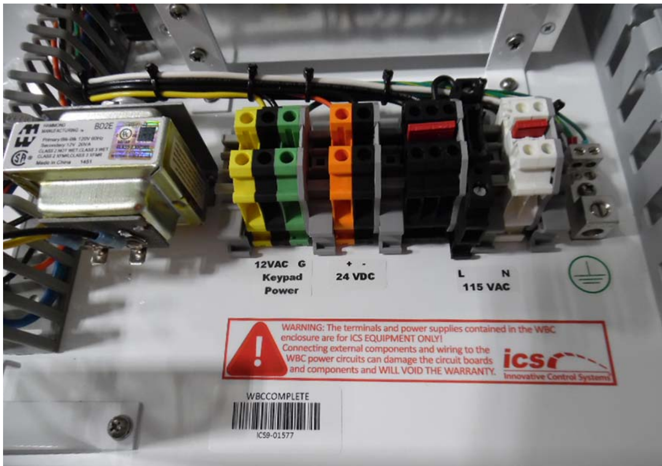
Figure 31. Warning label located below Tunnel Master® wbc Power Terminations
